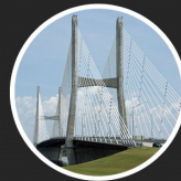
Bill Emerson Memorial Bridge Cape Girardeau, MO
