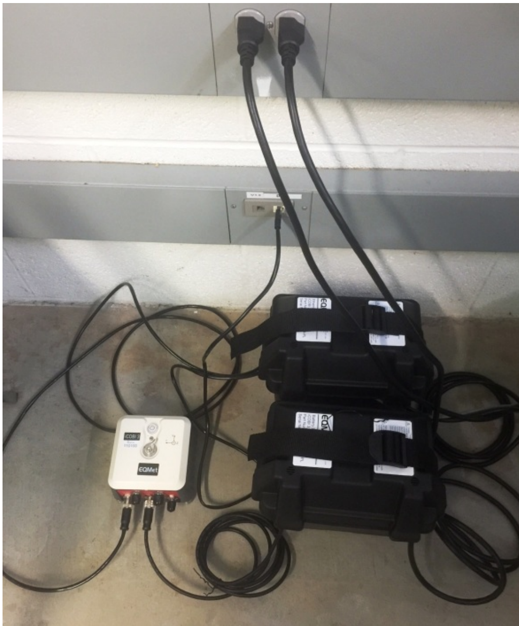
Figure 3.10: Typical installation of a Middle Accelerograph and Ethernet System
